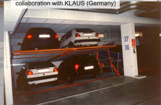
Multi-parking garages design in collaboration with KLAUS (Germany)
