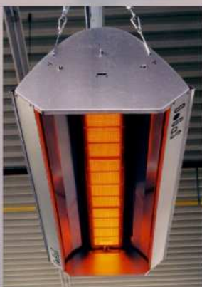
Heating system with GoGAS infrared burners for main production facility of Daugavpils driving chains plant. Year 2000
